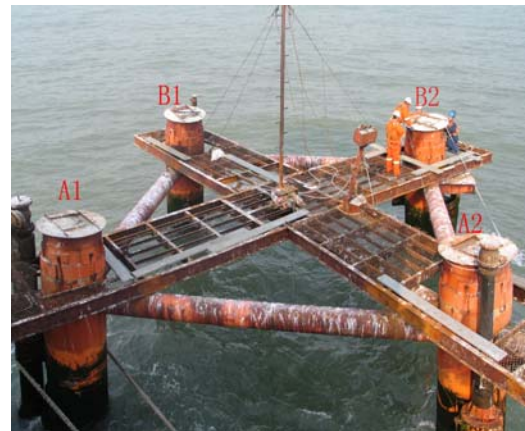
Fig. 1 The abandoned SZ36-1 SPM jacket
