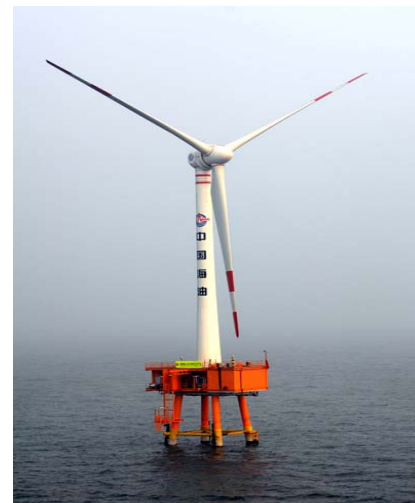
Fig. 2 The demonstrator project of wind turbine
